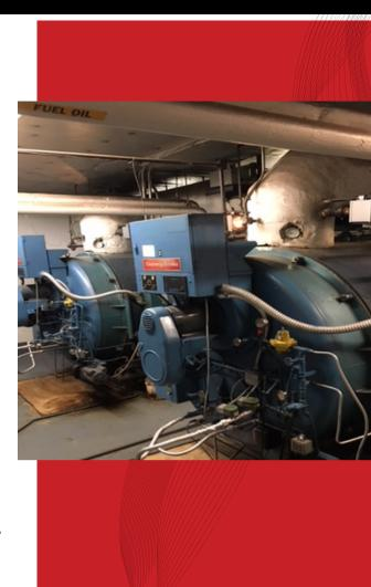
RBI is an integral part of the Midwest Courts' central operating system. RBI's domestic water heaters assist in eliminating storage which was originally planned for during the design phase. The compact size of the Futera XLF allowed installation to occur alongside demolation keeping the building fully operational for occupants.
